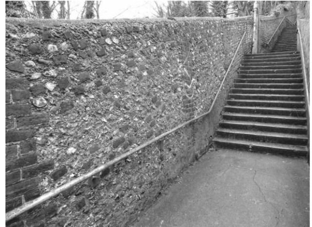
The flint and bits of brick walls on the cat creep – classic Brighton Bungaroosh building material. Bungarush is used in many Brighton houses, hidden behind plaster. It can make hanging a picture incredibly tricky. You either hit a flint and bend the nail, or start dislodging handfuls of loose lime mortar and pebbles. There is another length of bungaroosh wall where Crescent Road meets Princes Road.
