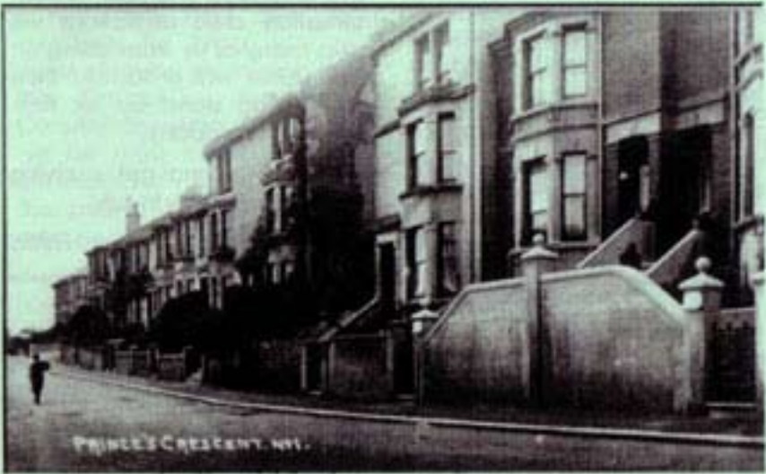
Princes Crescent around the turn of the last century, was one of the pictures shown by Jacqueline Pollard in her talk to the society. Number 85 had not yet been built. Note how none of the houses have their rendering painted - a feature widespread not just in Round Hill, but across Brighton.
