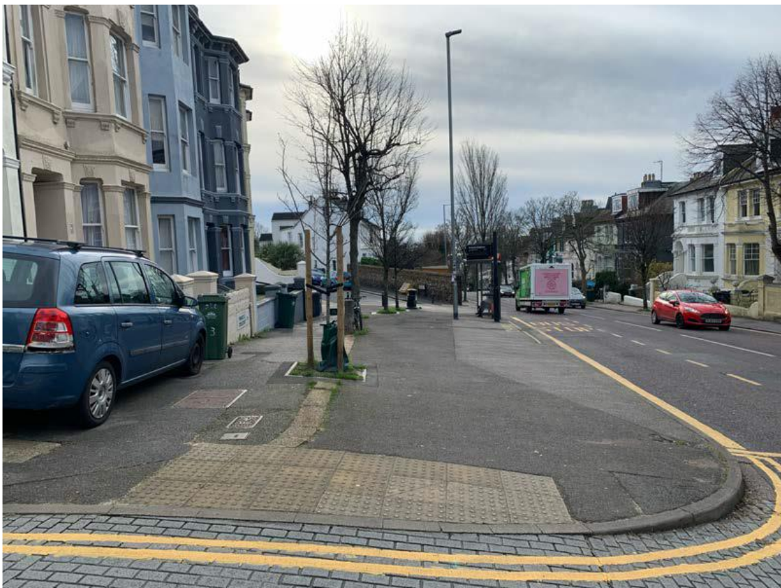
Figure 3. View of the Site from the junction with Round Hill Road
